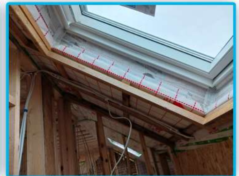
Velux roof light airtightness detail
