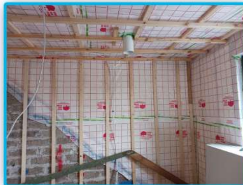
PHS Apollo 2 VCL Membrane PHS Argo Plus Sealing Tape PHS Modbau Window Tape
